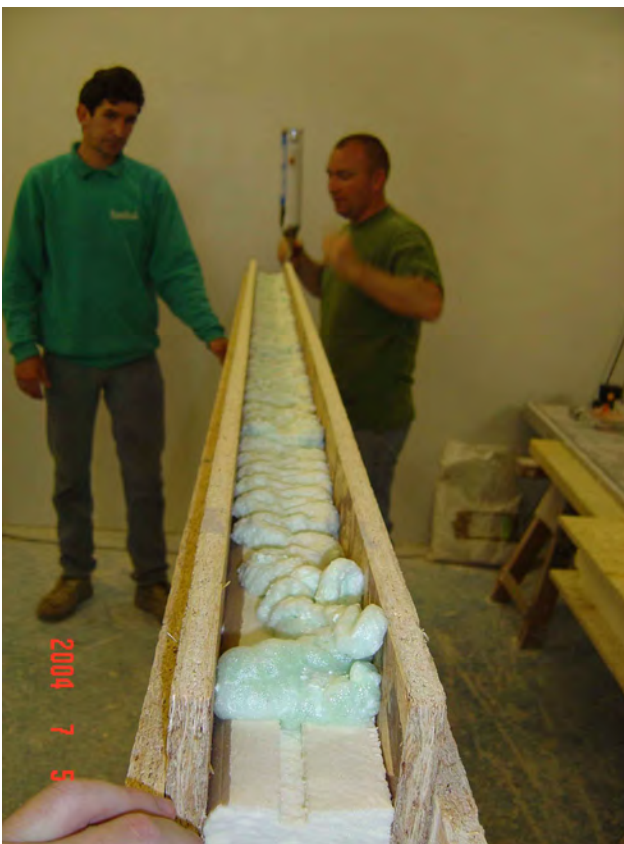
Photo 3 Applying the urethane expanding foam
