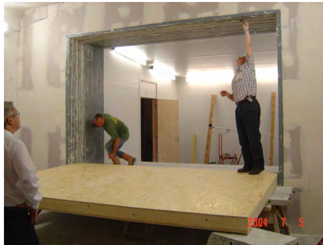
Photo 5 Assembled Kingspan Tek Partition
