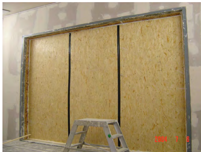
Photo 6 Kingspan Tek Panel System within test frame
